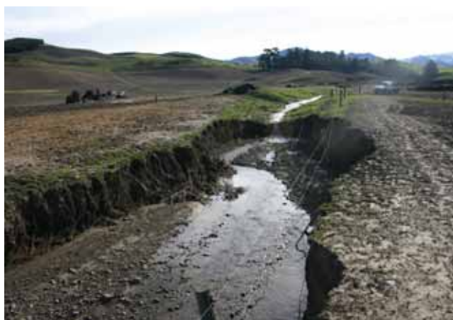
In this photo willows were completely removed leading to erosion.
